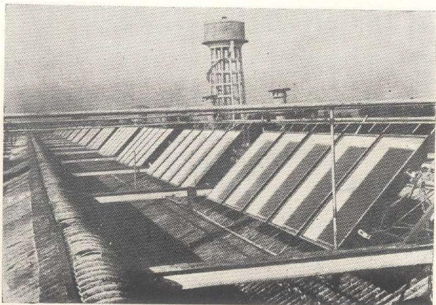
**Fig 9** An array of NPL-designed flat-plate solar collectors installed on a section of the Hardwar factory of Bharat Heavy Electricals Ltd.
